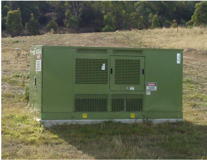
Padmount Substation
