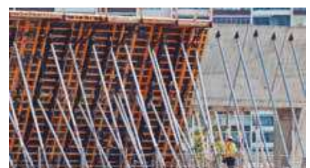
► Shoring in inclined walls
