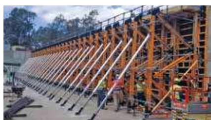
► Shoring in single-sided wall formwork
