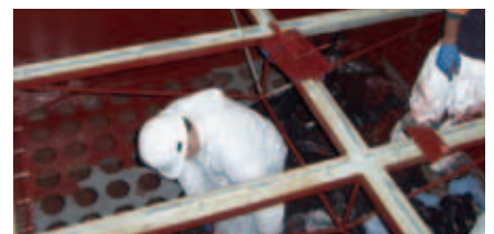
Applying LOCTITE® Nordbak High Temperature Brushable Ceramic
