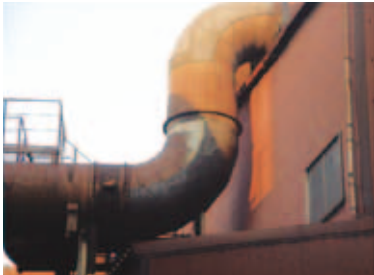
Plant pipe elbow, repaired with LOCTITE® Nordbak Pneu-Wear
